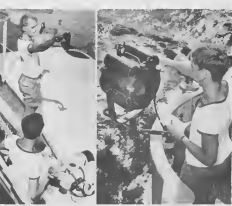
VISUAL SHIP to ship communications are made by semaphore and Minker. The position of two flags, left, indicates a letter. Flashing light from lamp, right, indicates letter. COMUNICACION VISUAL di bapor pa bapor ta worde haci cu semafoor y luz. Posicion di e dos banderanan, rubes, ta indica un letra. Luz brillando, banda drechi, ta indica letra.
